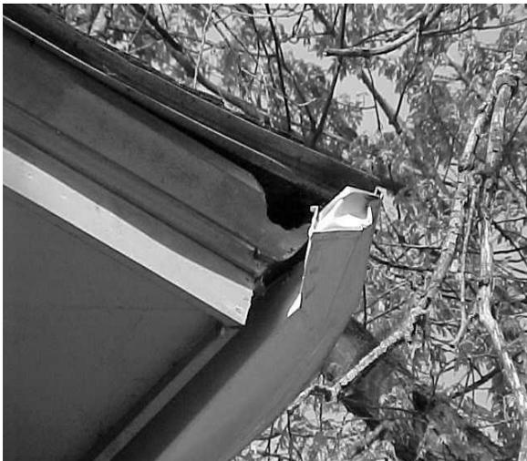
**Figure 2.** Tree squirrel hole in a soffit.
