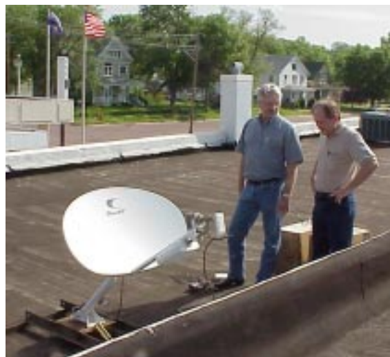
Jim Emal, right, and Terry Bockstadter, NU members of the Technologies Across Nebraska Partnership, in spring 2001 helped install Cooperative Extension's first nationwide two-way, high-speed satellite Internet system at the extension office in Fairbury.
